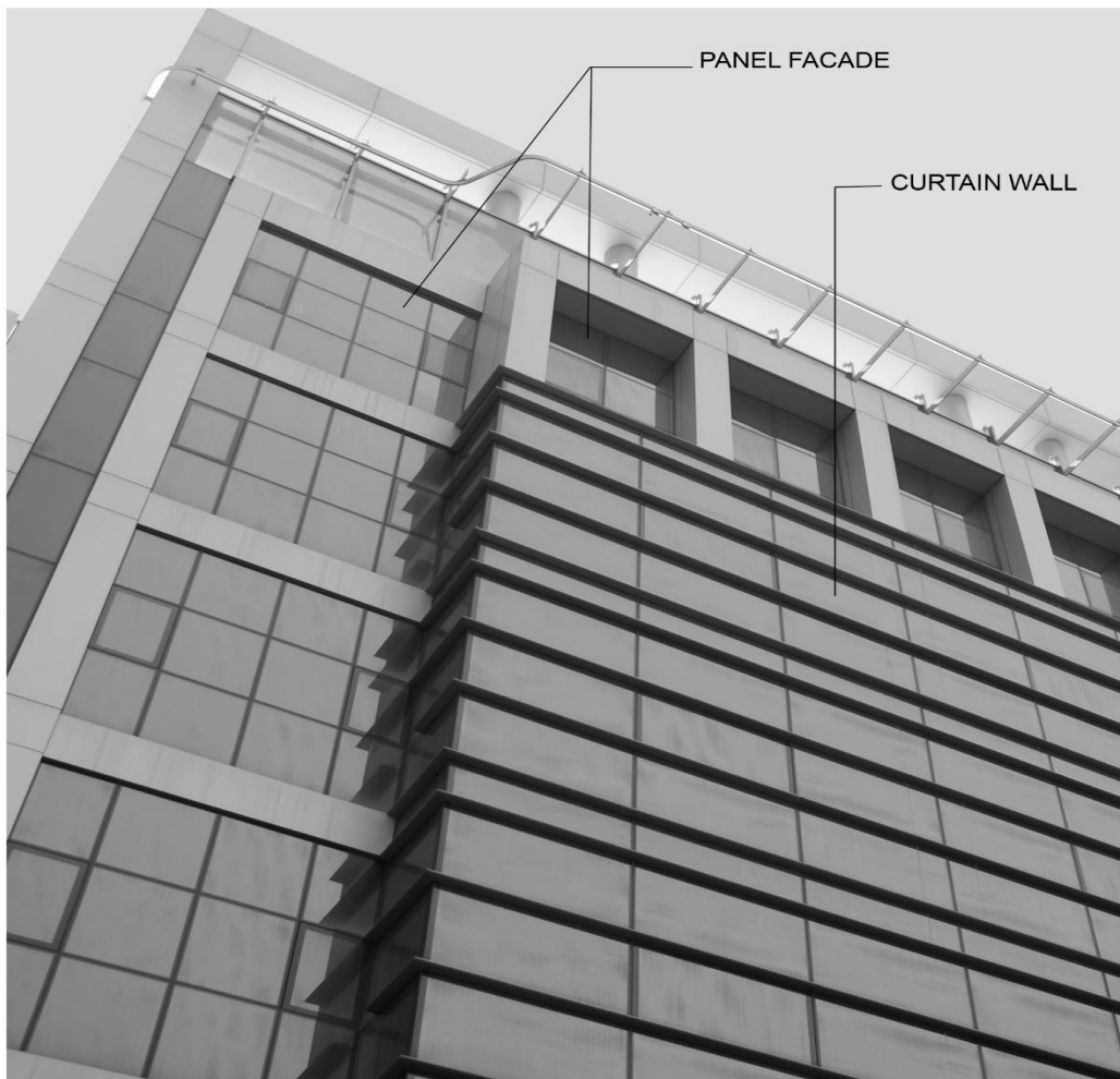
Image 02 Curtain wall and panel façade
